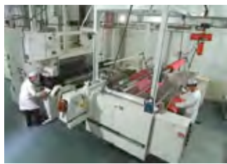
Argotec extrusion line in hard-walled cleanroom
