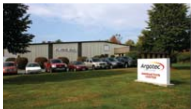
Flat-die and blown-film lab lines and hard-walled clean rooms enhance the Argotec Innovation Center
